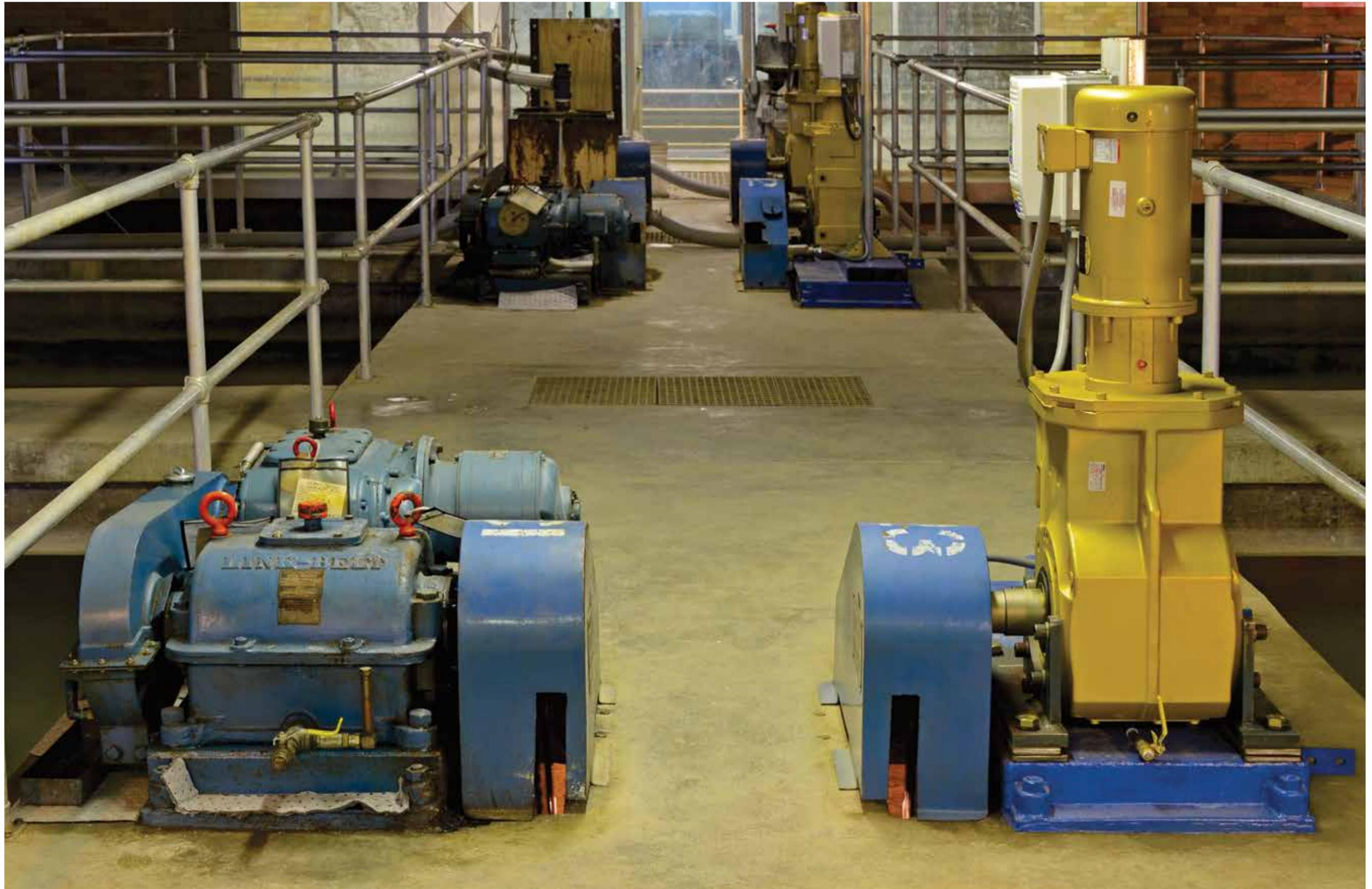
Aging mechanical variable speed drives, pictured on the left, are being replaced with a high-performance, energy efficient Baldor•Dodge® Quantis® Gold solution that includes a Dodge Quantis right-angle helical bevel (RHB) reducer with a Baldor•Reliance® Super-E® premium efficient motor, along with a Baldor drive. Plant officials say this system allows them to precisely control the speed of the submerged paddles in the treatment basins.
